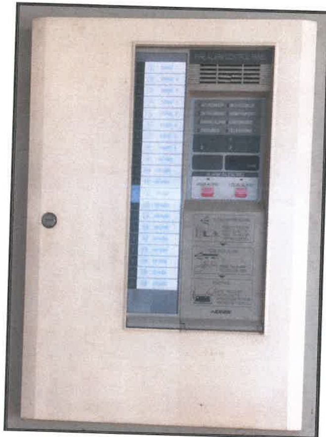
FIRE ALARM CONTROL PANEL (FCP.)
